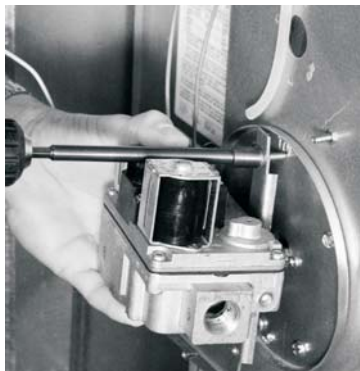
FIGURE 3: Gas Valve Removal
