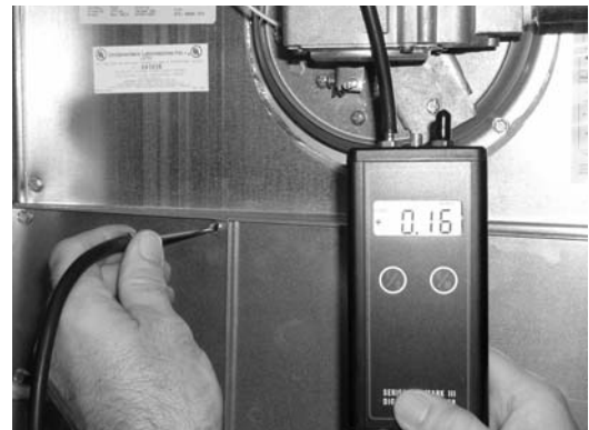
FIGURE 20: Measuring supply static pressure
