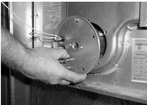
FIGURE 4: Burner Assembly Removal
